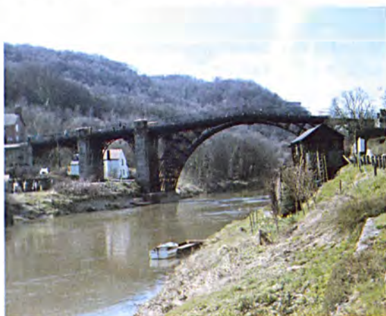
The World's first Ironbridge, Ironbridge, Shropshire (erected 1779).
