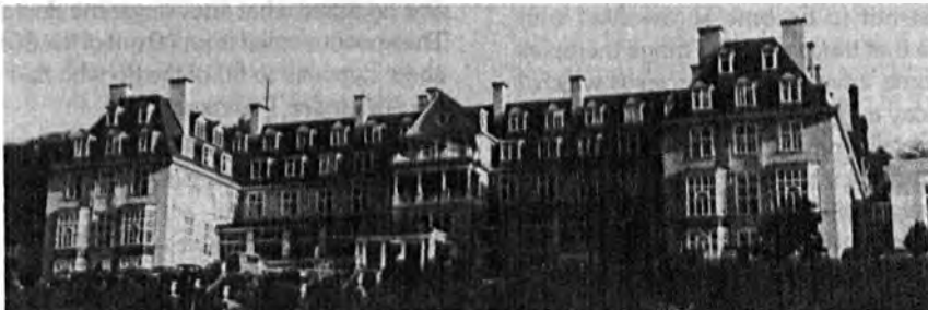
Peebles Hydro Hotel
